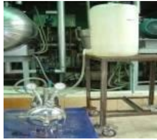
Figure 6. The pressurized tank connected with solution tank.
